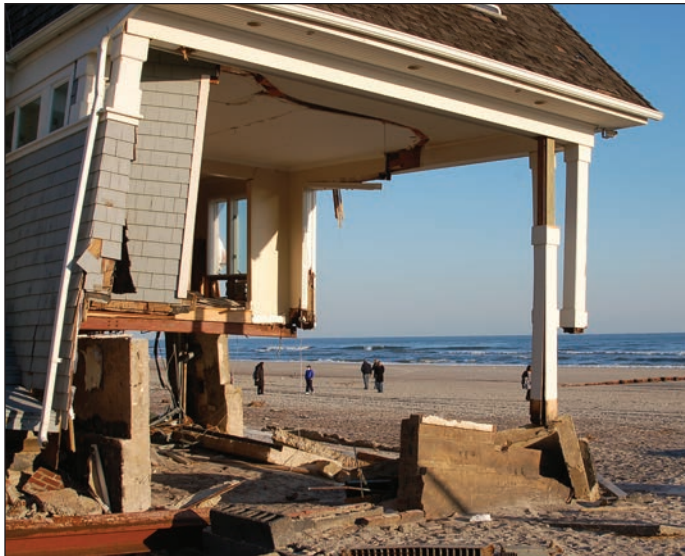
Figure 6: Wave, storm surge, and erosion damage to oceanfront house at Rockaway, NY
