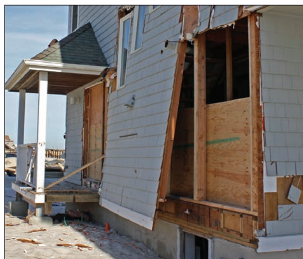
Figure 1: Back wall failure due to flood level above the lowest floor of a house in Ortley Beach, NJ
